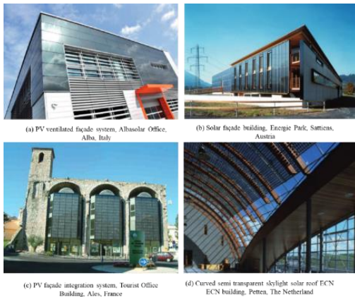
Figure 4. Architectural and design-oriented solar PV integrated buildings in Europe (Heinstein et al., 2013)
