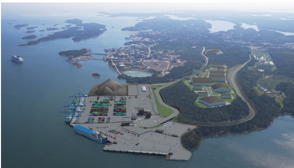
Figure 1. Norvik multi-terminals seaport: Ro-Ro and containers terminal
